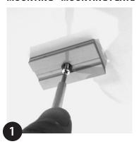
Check product/plate orientation and cable grommet clearance from mounting surface. Mark position of plates (supplied with the preinstalled sliders – 2 per metre).
